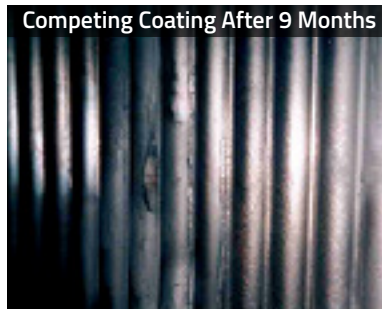
Competitors coating shows damage from erosion requiring repair.
