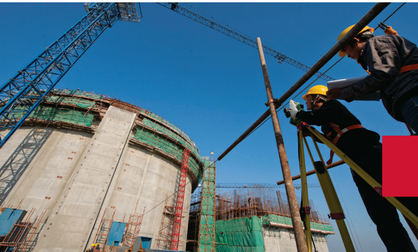
Fuqing nuclear power station under construction in China.
