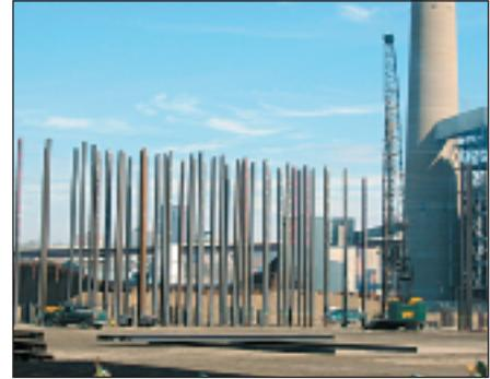
While a crane positioned a second 50-foot beam vertically over the first already in the ground, another team tack welded the two beams end to end in a butt weld. Then, a third team finished the job, first by welding three passes on one side of the H-beam joint. Then, the same team arc gouged the joint backside and welded three passes there as well.
