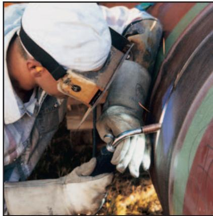
pipeline could handle the pressure range of the Gulfstream system. Pipe is coated with a Fusion Bond Epoxy (FBE) on both the interior and exterior, and a majority of the pipe is also concrete coated for buoyancy control.
