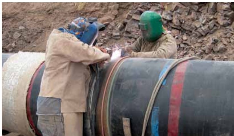
The self-shielded flux-cored wires, Pipeliner® NR-207s and 208s, are often the simplest wire solution. There is no stub loss, no gas shielding is required and these wires can be used to weld pipe grades of up to X80.
